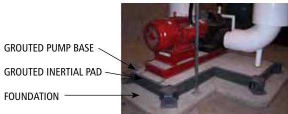
Typical Inertial Pad Installation Figure 32
